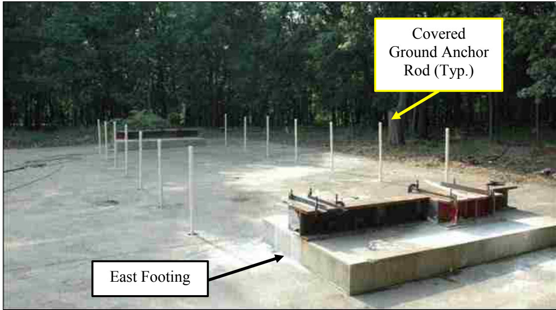
Figure 3.24: Installed ground anchor rods covered by plastic pipes (Sause et al., 2009)
