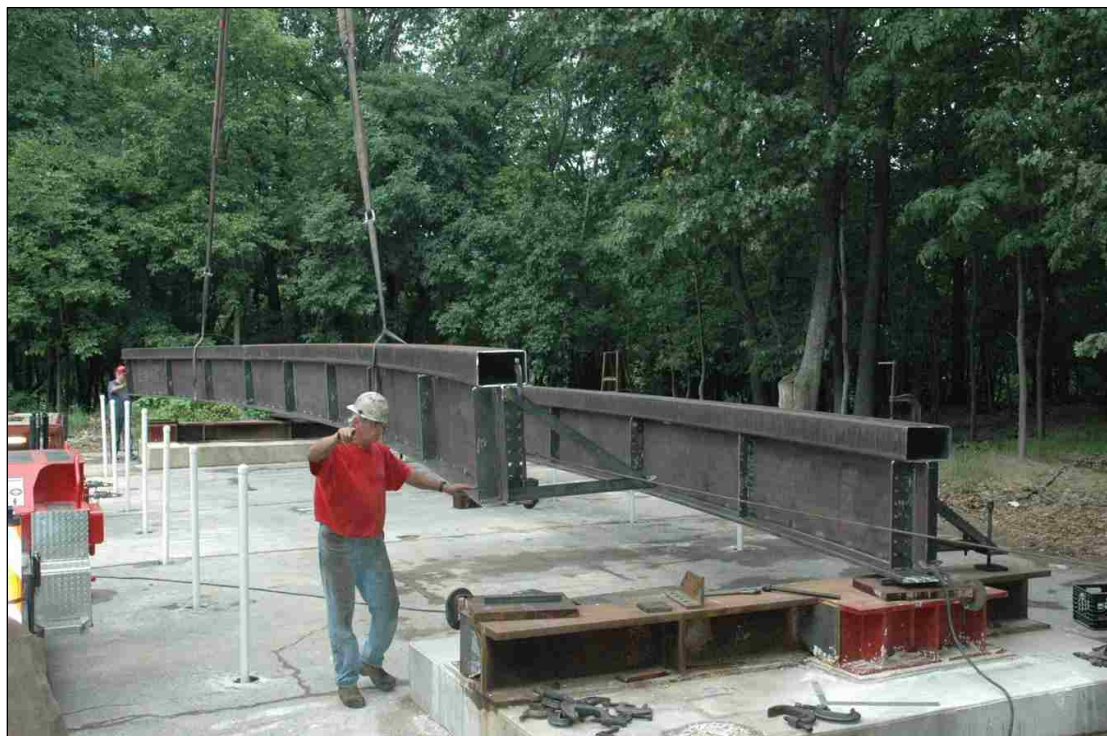
Figure 3.20: Erection of test specimen (Sause et al., 2009)
